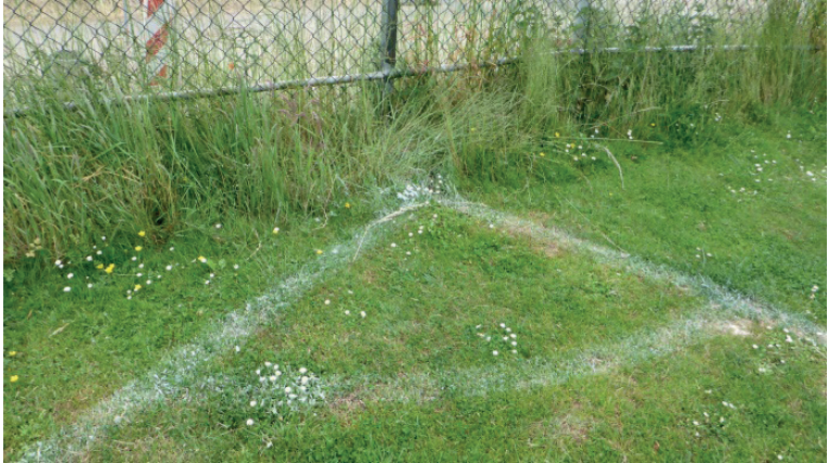
Minimum safety distance and unobstructed distance are not maintained (cf. DIN 18035, part 1)
