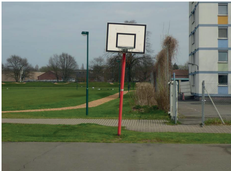
Crooked streetball installation. This may reduce stability.
