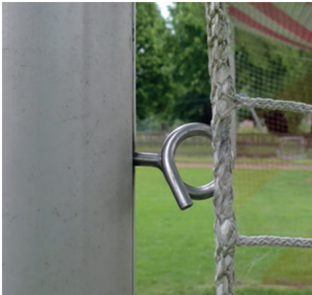
DIN EN 748 does not permit open metal hooks.
